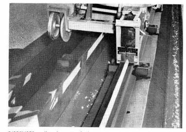
DISPENSER rolls along track laying continuous bead of braking
